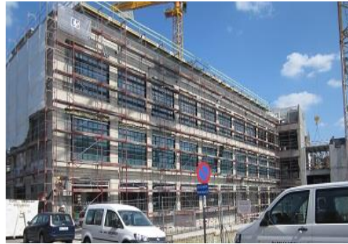
Sprayed OMNIGUARD film as protection of the inside of windows during construction works, till the end of the jobsite.
