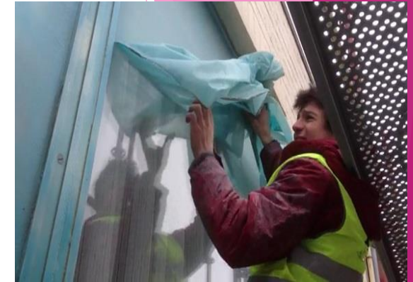
OMNIGUARD served as a protection of the aluminium windows
