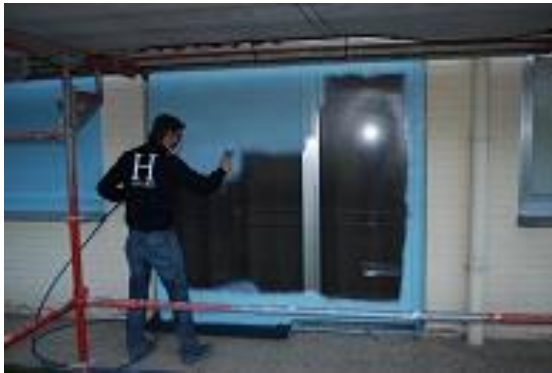
Sprayed film as protection of the outside of the windows during facade renovation works
